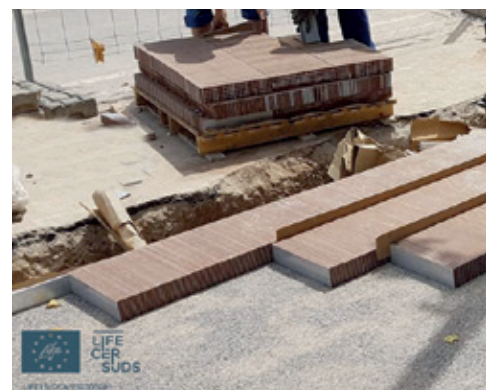
CERSUDS PROJECT: DEMONSTRATOR - INSTALLATION OF CERAMIC MODULES
